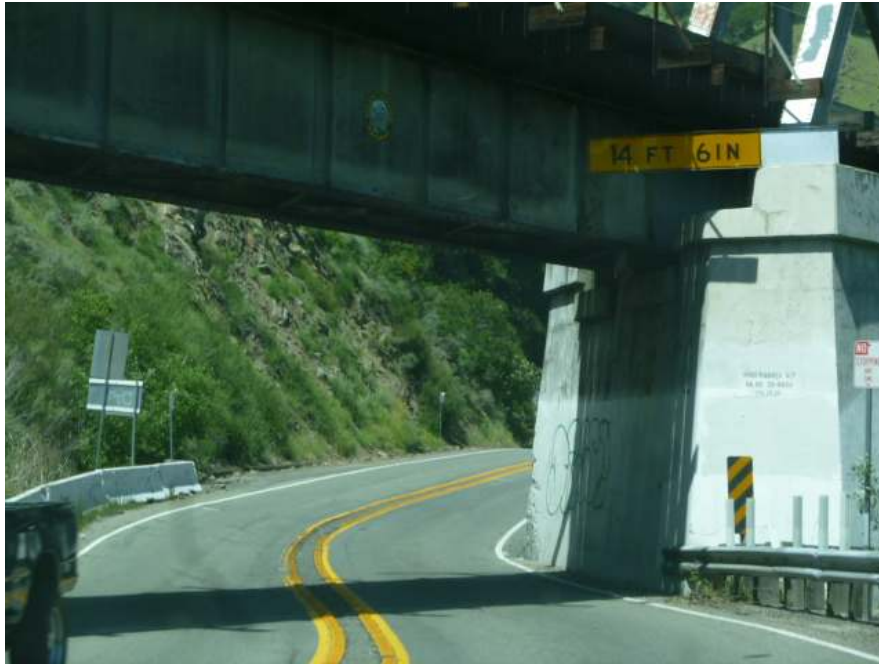
View of Rosewarnes Underpass traveling eastbound
