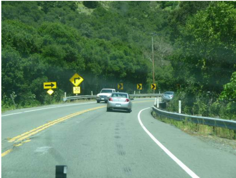
Metal beam guard rail at low height and without appropriate end treatment (east approaches to Alameda Creek Bridge)
