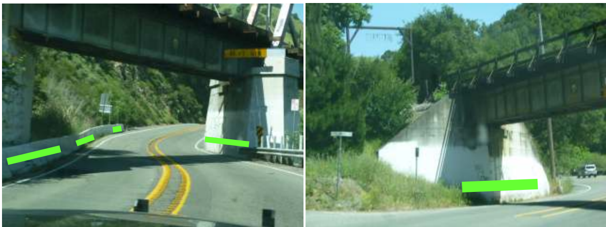
Traveling Eastbound at Rosewarnes Underpass (Left Picture) and at Farwell Underpass (Right Picture)
