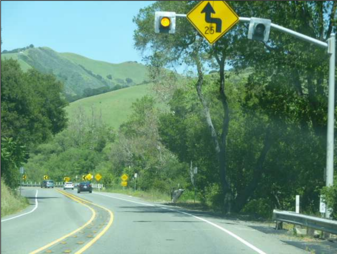
Traveling east approaching first curve at the Rosewarnes Underpass
