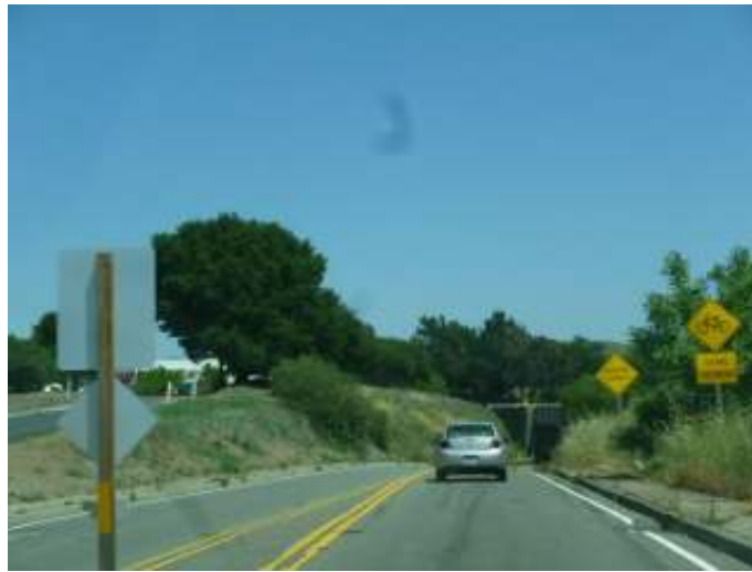
Traveling eastbound approaching the Silver Springs Underpass
