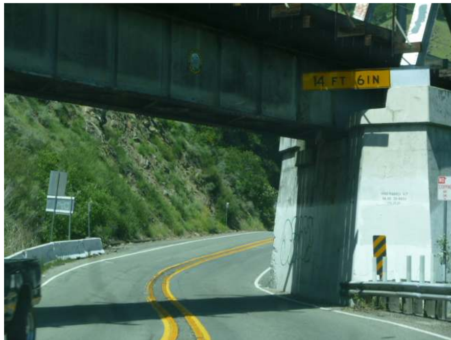
View of Rosewarnes Underpass traveling eastbound
