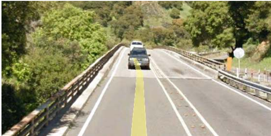
Looking eastbound across the Alameda Creek Bridge BOH
