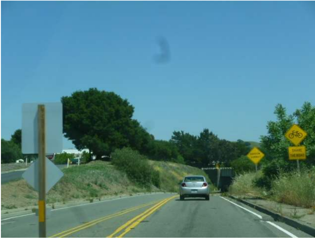
Traveling eastbound on SR 84 approaching Silver Spring Underpass
