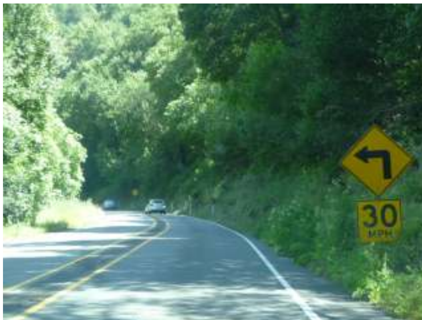
Traveling eastbound approaching 30 mph curve between the two bridges
