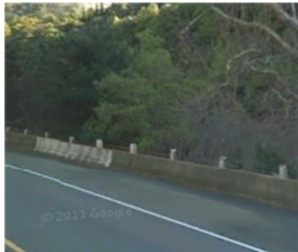
Barrier east of Farwell UP along eastbound lanes
