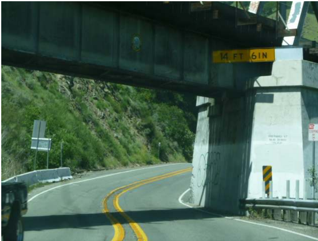
View of Rosewarnes Underpass traveling eastbound
