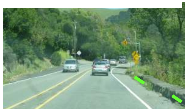
Rock wall preceding Rosewarnes Underpass
