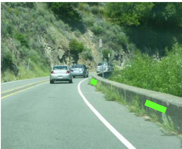
Concrete/Rock Wall (east of Rosewarnes Underpass)
